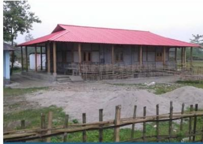
Eg. The KEBA Sub Center Building in Arunachal Pradesh
