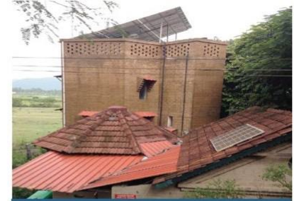
Eg. Solar System Design at Tribal Hospital, Tamil Nadu
